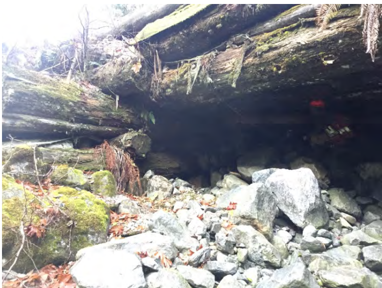
Right Bank Abutment when facing downstream
