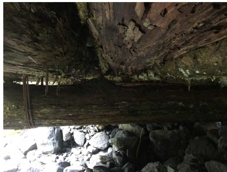
Needle beam not functional
