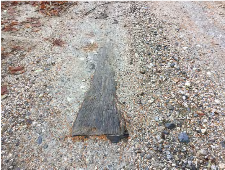
Stringers at surface
