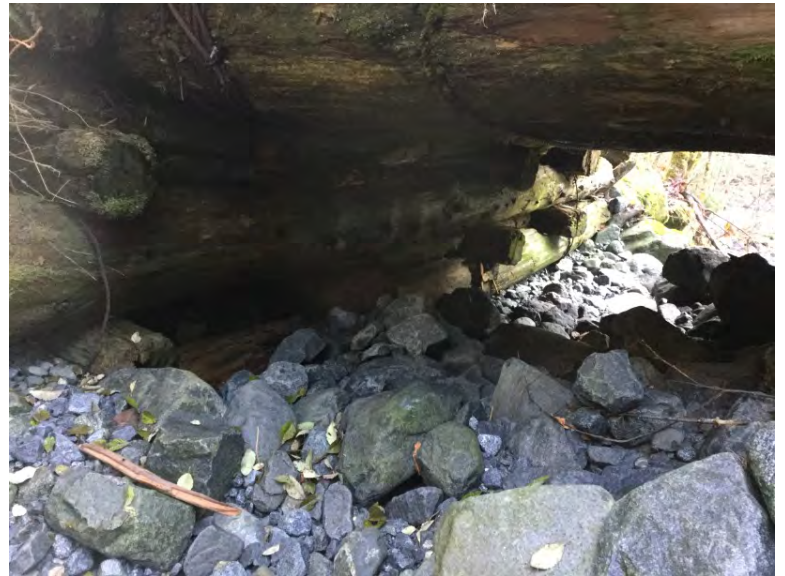
Left Bank Abutment when facing downstream
